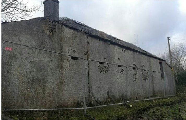
Unit two (north elevation)
