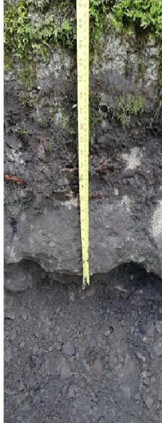
Unit one (foundation)
