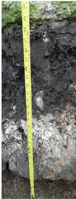
Unit two (foundation)
