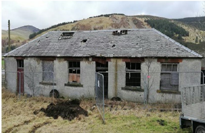
Unit two (south elevation)
